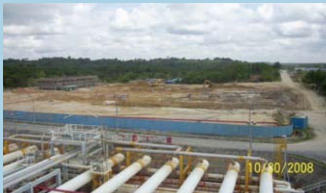
Latest View of PCK - 6 Zone 5 Construction Area
