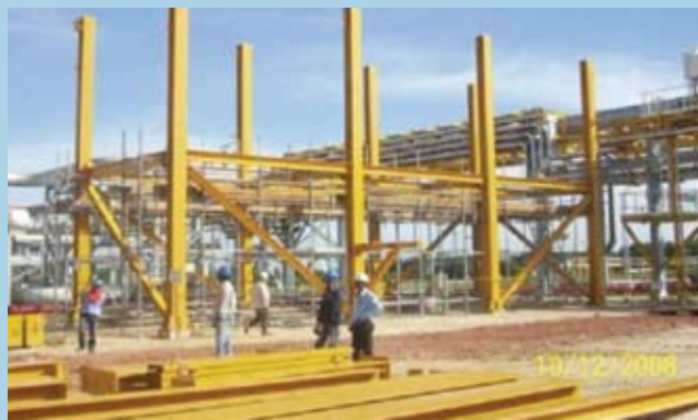
Erection Sensitive Well Flaring
