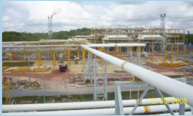
Latest View of PPA Main Pipe Rack Area
